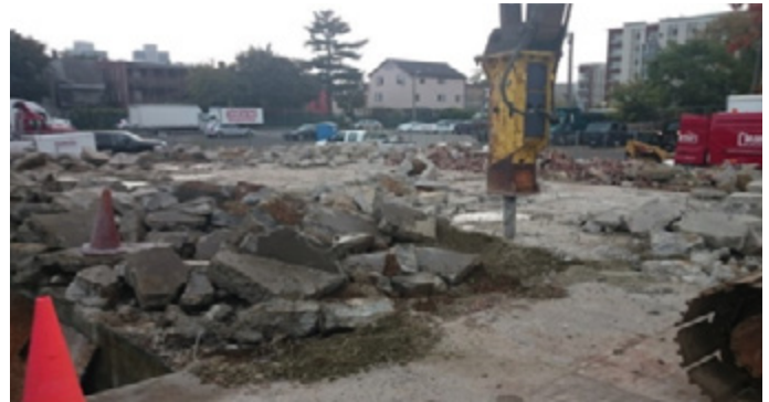
View of concrete slab demolition
