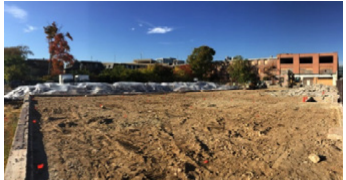
View of strategic excavation
