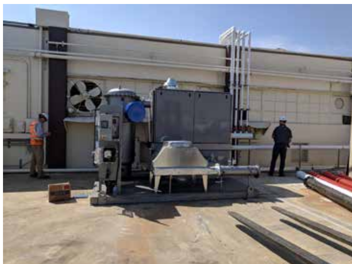
View of permanent Soil Vapour Extraction system – former CMI site
