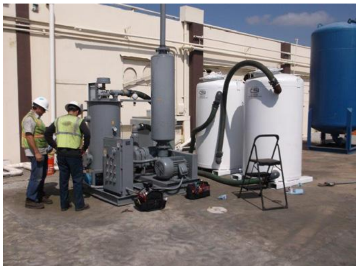
Interim Soil Vapor Extraction System View - Former CMI Site
