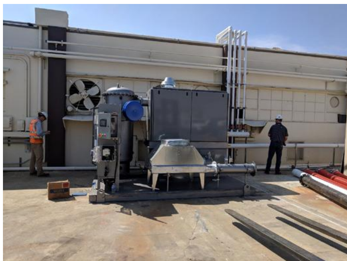
View of Permanent Soil Vapor Extraction System- Former CMI Site
