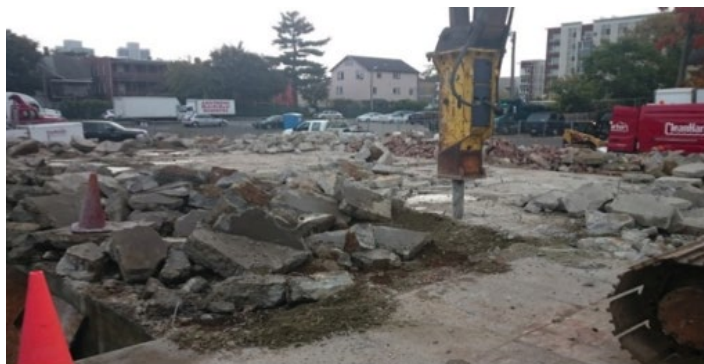
View of concrete slab demolition
